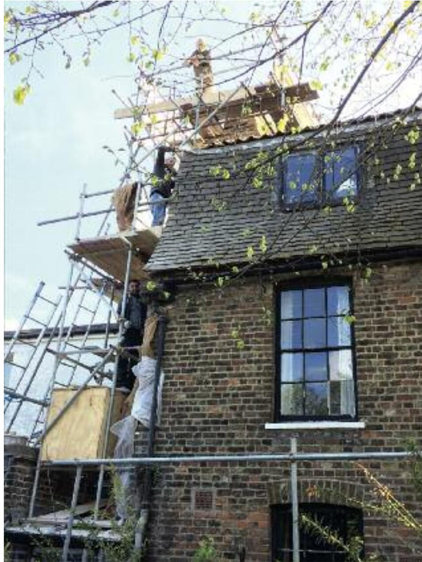
Left: Scaffolding in place, 'the battle of the bulge' begins. Below left: The huge bulge is shored up as a matter of urgency by scaffolding constantly adjusted to accommodate its horrifying contours. Below: Exposed inner leaf masonry
